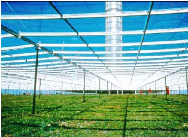
Fig. 6 Glass roof of the prototype plant at Manzanares, Spain
